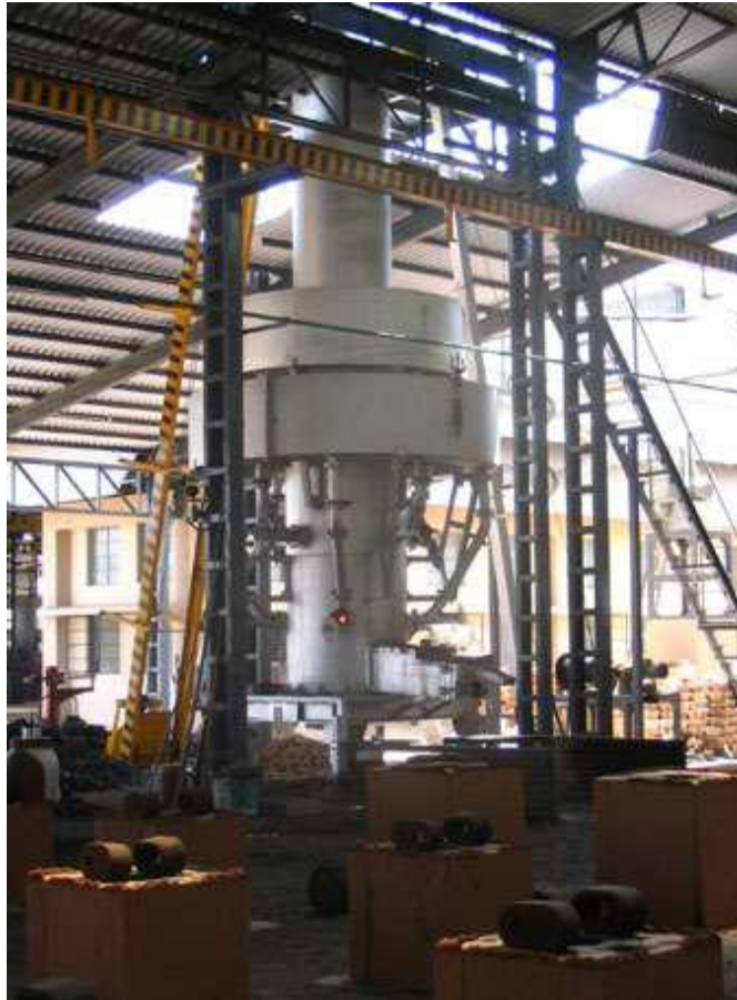
Figure 2: Divided Blast Cupola Furnace
